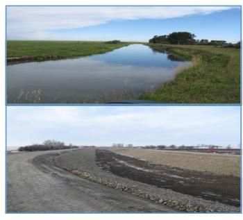
This project is a continuation of the rehabilitation of the Secondary A Canal System and starts at Highway 24 ending close to the Cairnhill Spillway. The canal design increases the canal capacity, improves accessibility, and eliminates seepage. This reach of canal is in the current Seepage Control Plan. Caliber Systems Inc. is the main General Contractor on this project.
